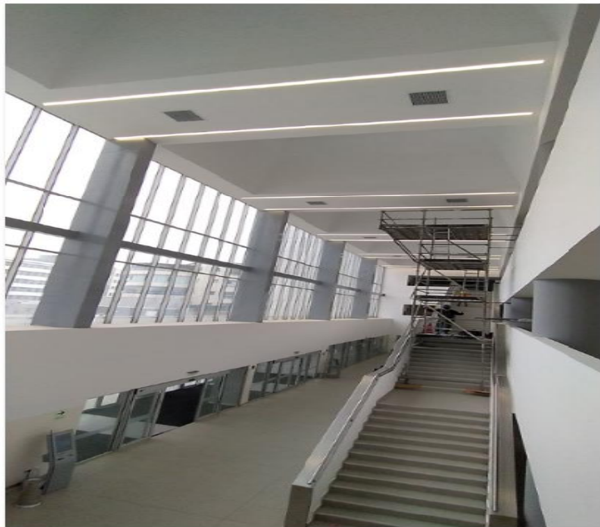
Figura 68 Luminarias Patos-Line Led 32 W 4400 Lm plx 840/linia-EL
