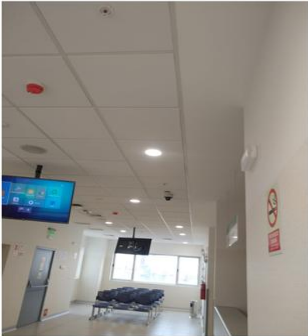
Figura 62 Luminarias tipo Beryl Led 10/15/24/35W
