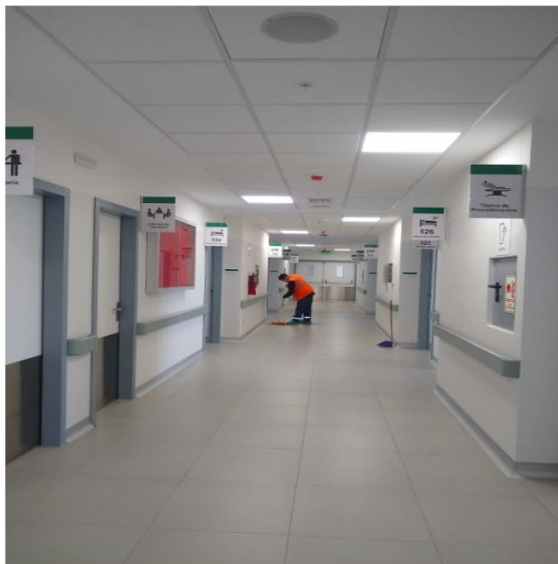
Figura 63 Luminarias Panel EMP Led 40W (605x605) 4000K
