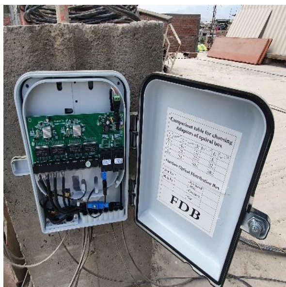
Fig. 9. Caja NAP (Network Access Point)
